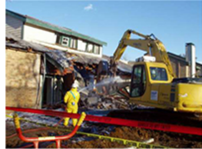
The "wet method" of asbestos removal in Ft. Worth.
