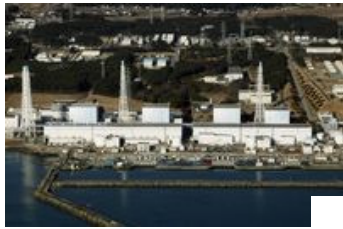
An aerial view shows the quake-damaged Fukushima nuclear power plant in the Japanese town of Futaba, Fukushima prefecture on March 12, 2011. (STR/AFP /Getty Images/Getty)
